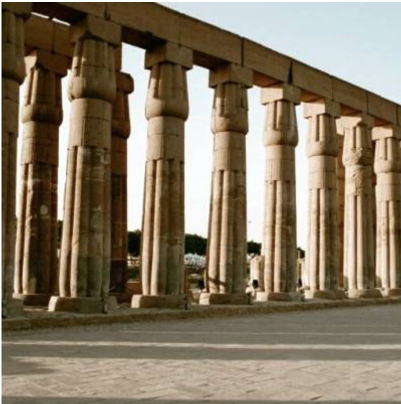
Fig. 7. Columns in sun court of Amenophis III.
