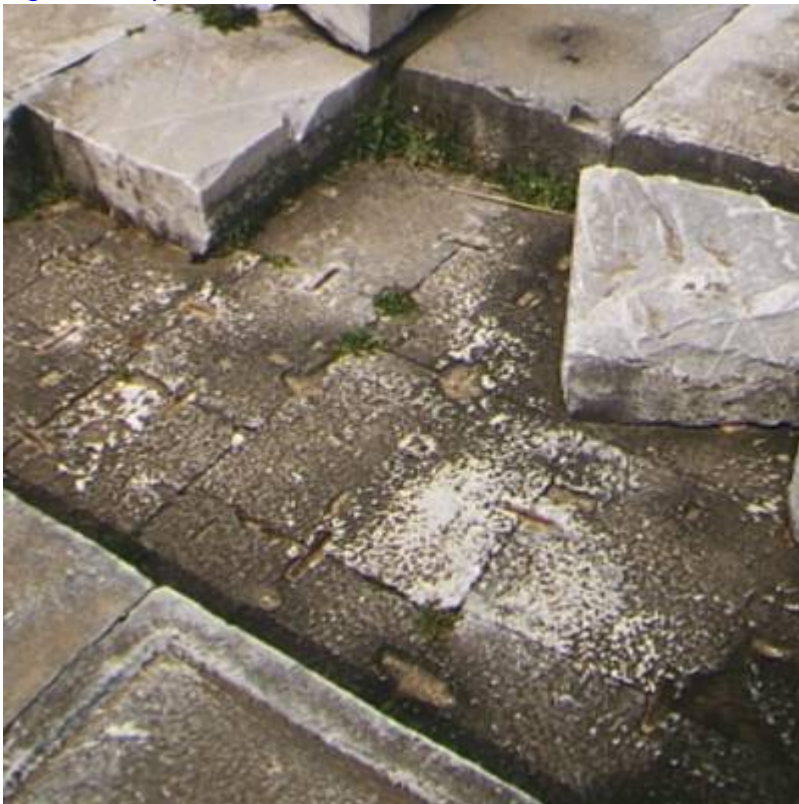
Fig. 8. Temple of Athena, paving anchor detail.
