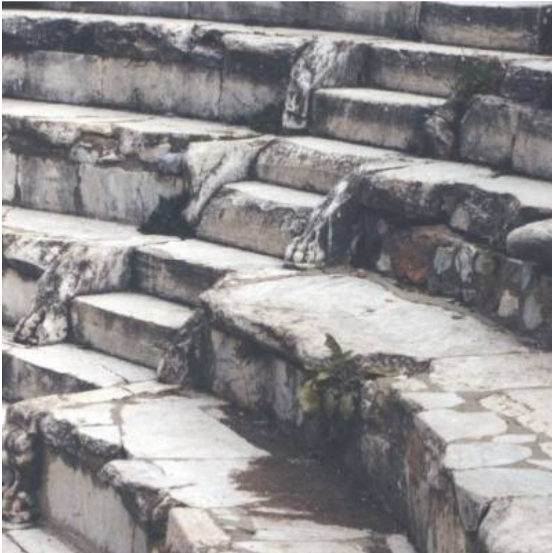
Fig. 5. The Odeion, noted detail at stairs.
