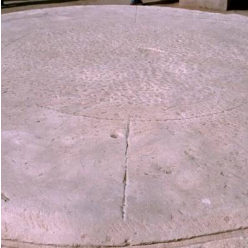
Fig. 1 Column base showing masons guide lines.
