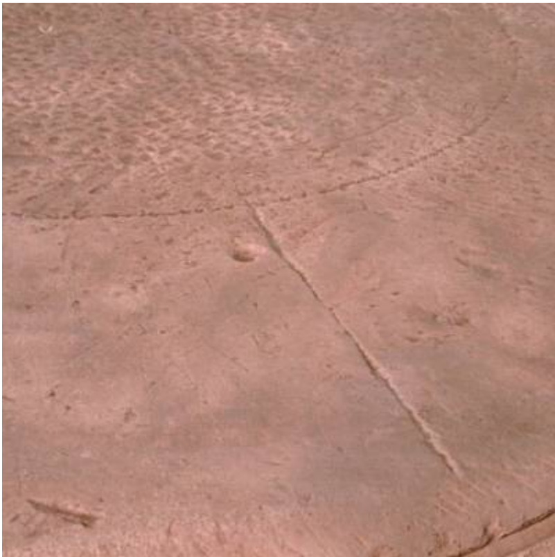
Fig. 2. Column base showing masons guide lines.
