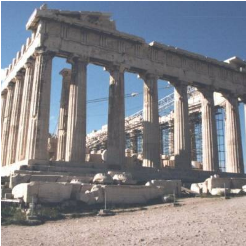
Fig. 4. View of eastern facade of the Parthenon.
