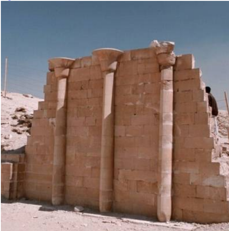
Fig. 12. House of the South, papyrus head and stalk pilaster.
