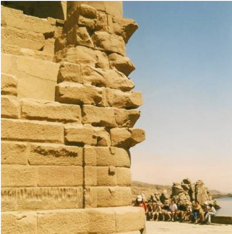
Fig. 13. Unfinished wall corner Kiosk of Trajan.
