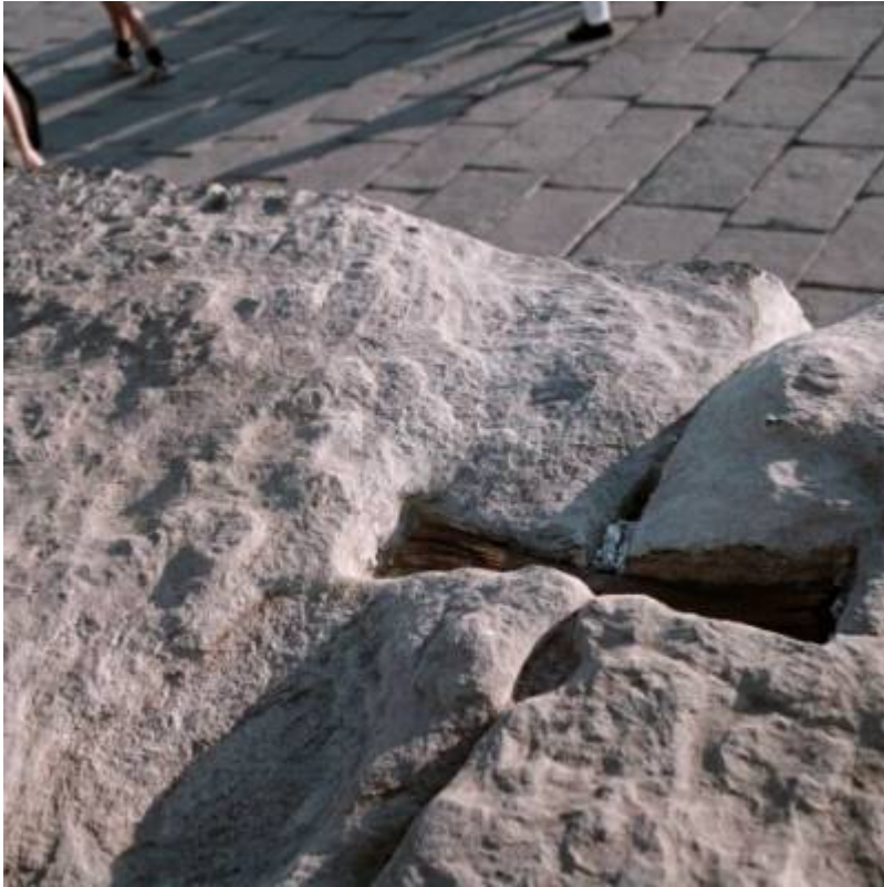
Fig. 10. Original wood dovetail in wall of Kom-Ombo Temple.
