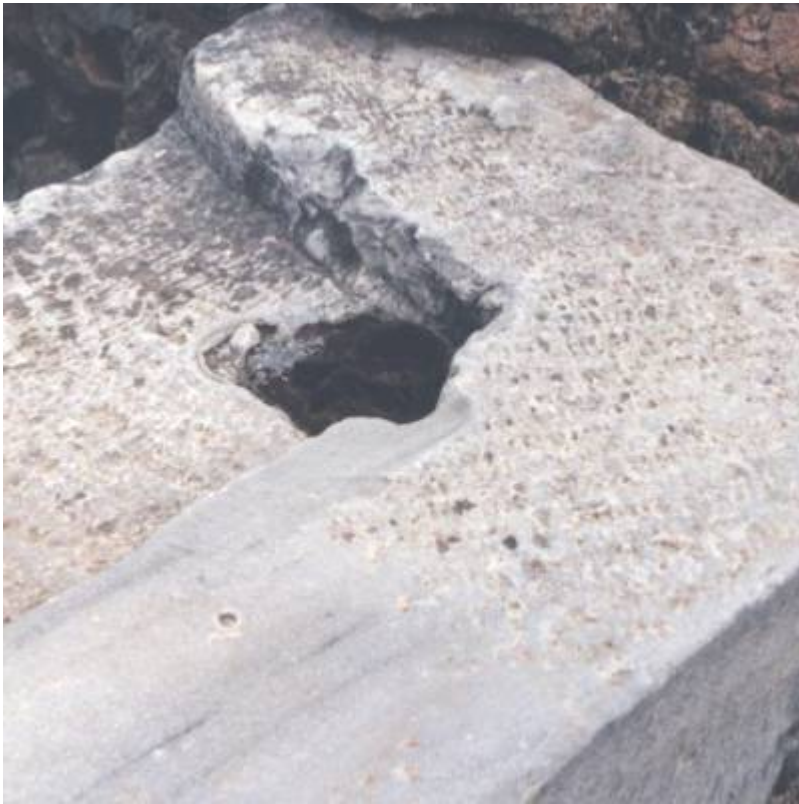
Fig. 7. Stone anchor detail.
