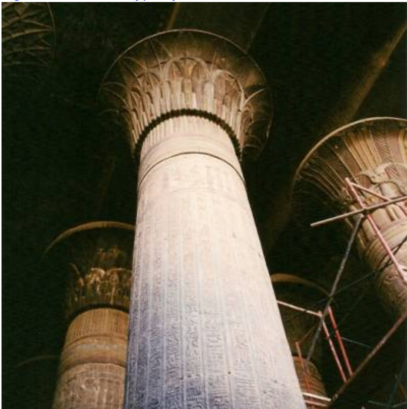
Fig. 6. Detail of column capital.
