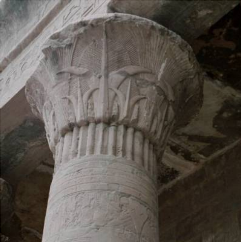
Fig. 6. Column capital detail from peristyle court.
