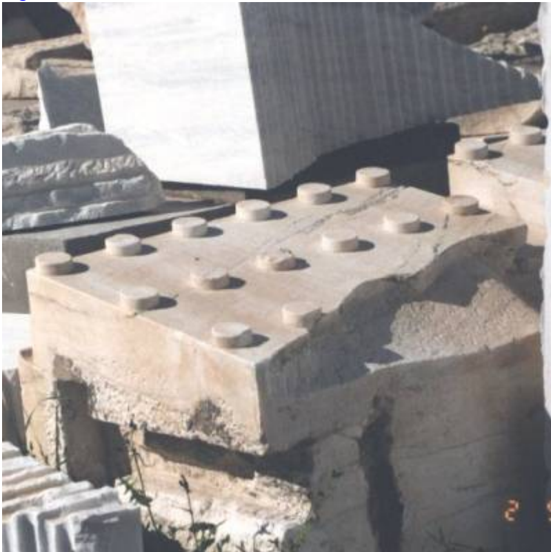
Fig. 8. The Parthenon, details of the mutule.
