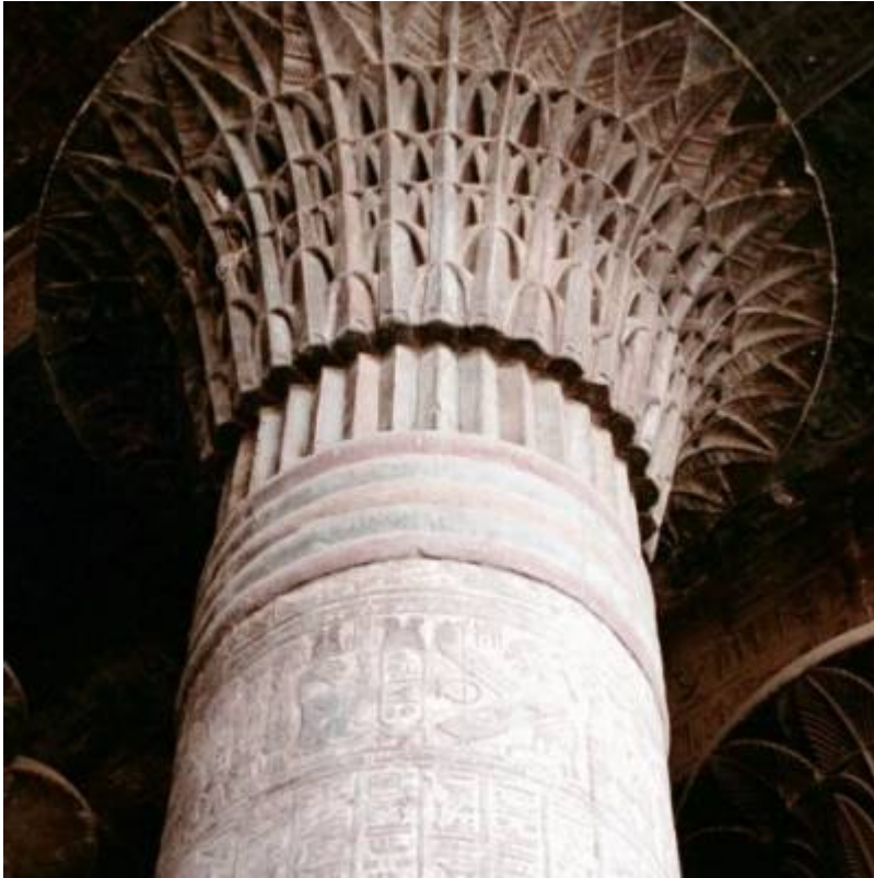
Fig. 7. Detail of column capital.
