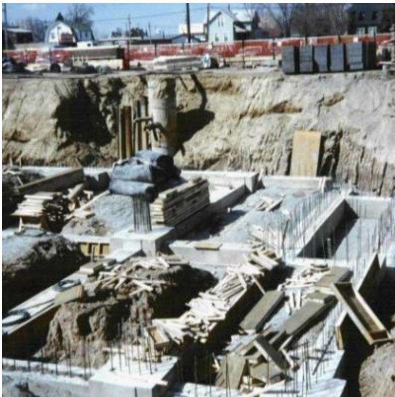
Fig. 20. Foundations - pier caps and grade beams.
