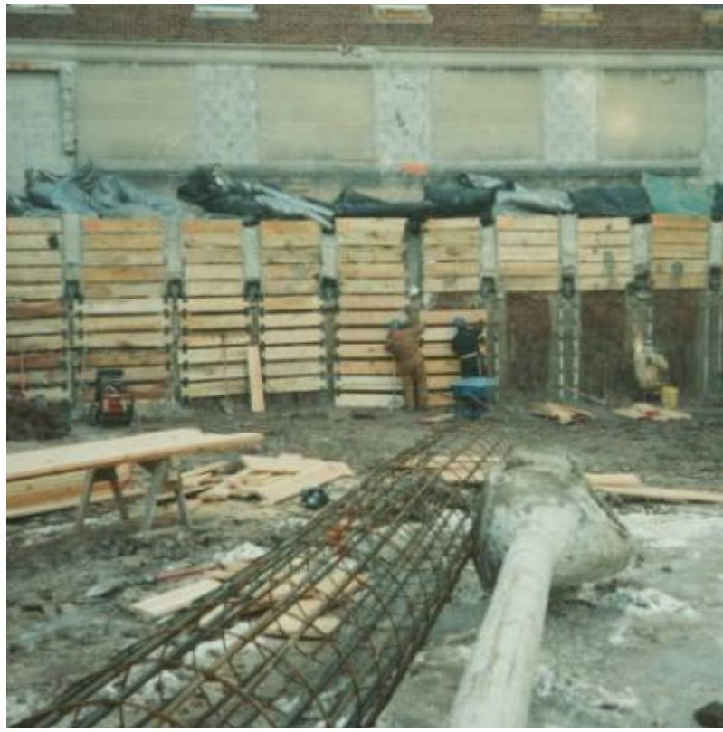
Fig. 4. Excavation and installation of earth retention system.
