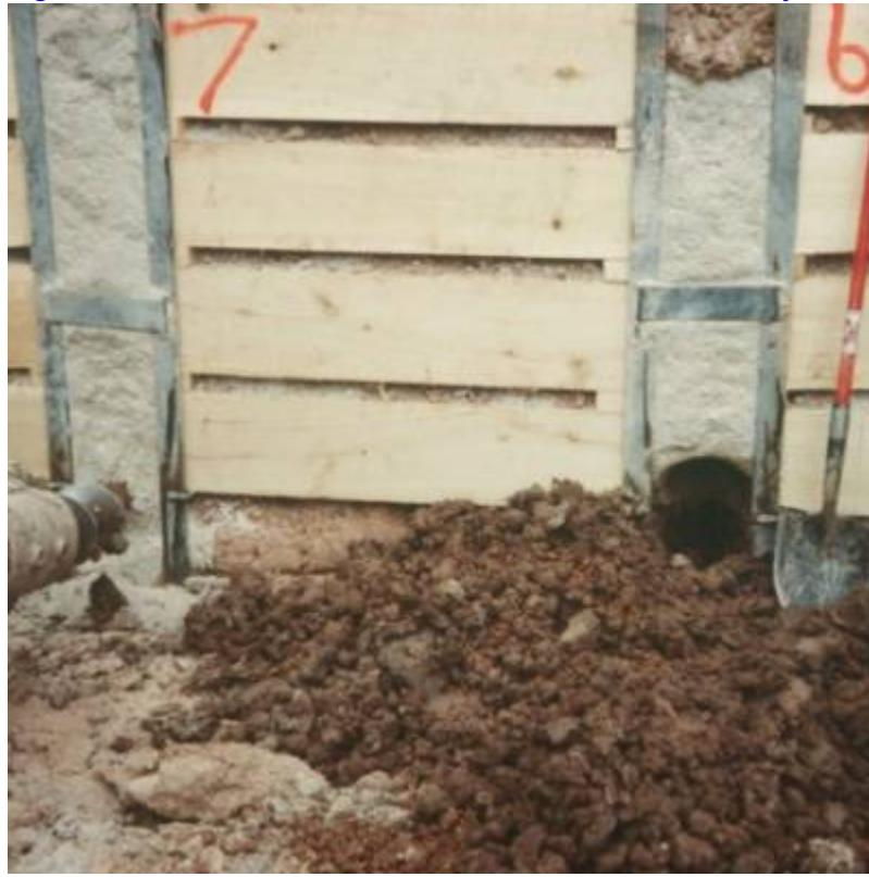
Fig. 5. Installation of soldier beam earth retention system.
