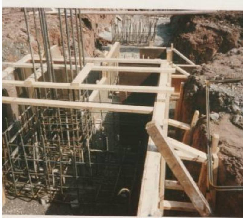
Fig. 18. Foundations - pier caps and grade beams.
