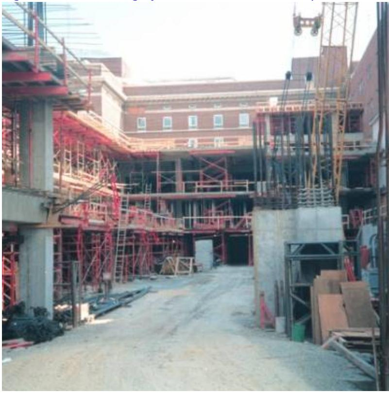
Fig. 23. Concrete framing systems - beam and slab and flat slab with drops.
