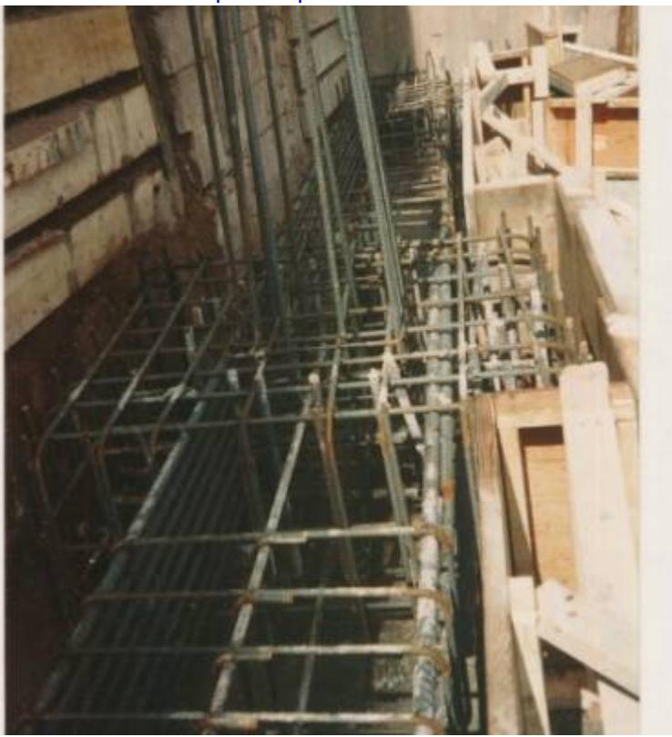
Fig. 17. Foundations - pier caps and grade beams.
