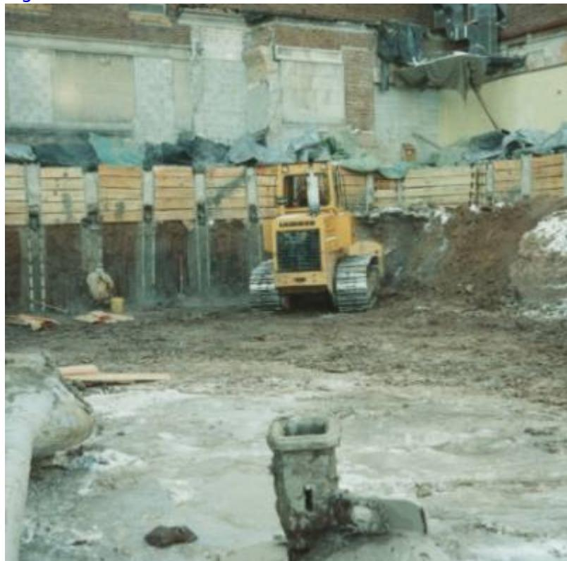
Fig. 3. Excavation and installation of earth retention system.
