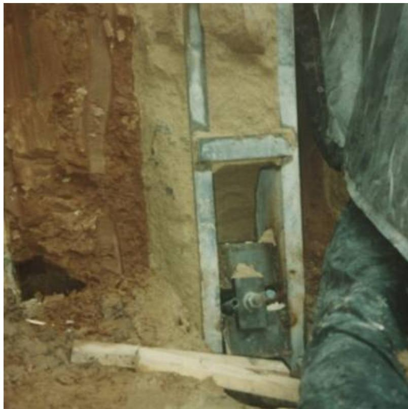
Fig. 6. Installation of soldier beam earth retention system.
