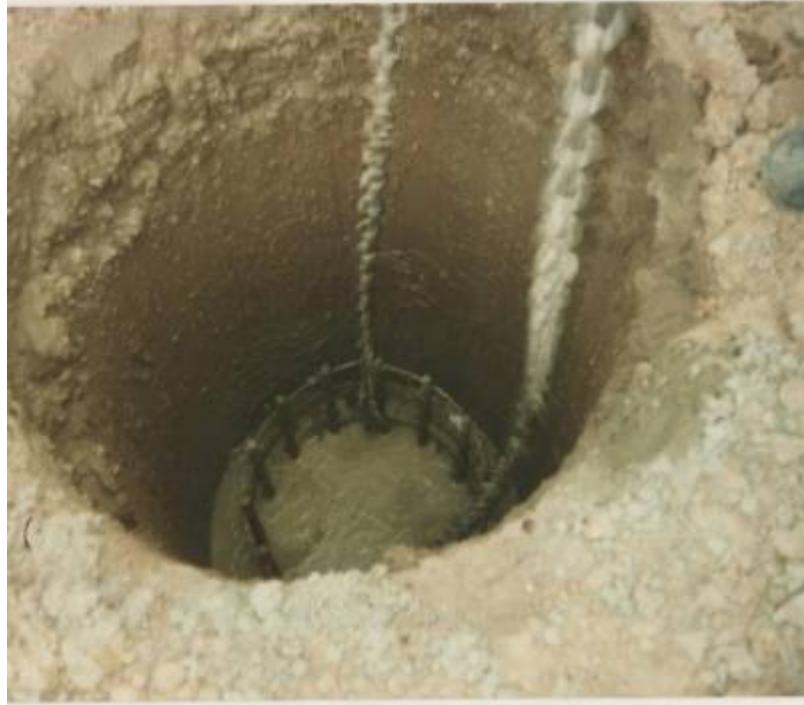
Fig. 15. Drilled pier after concrete has been placed.
