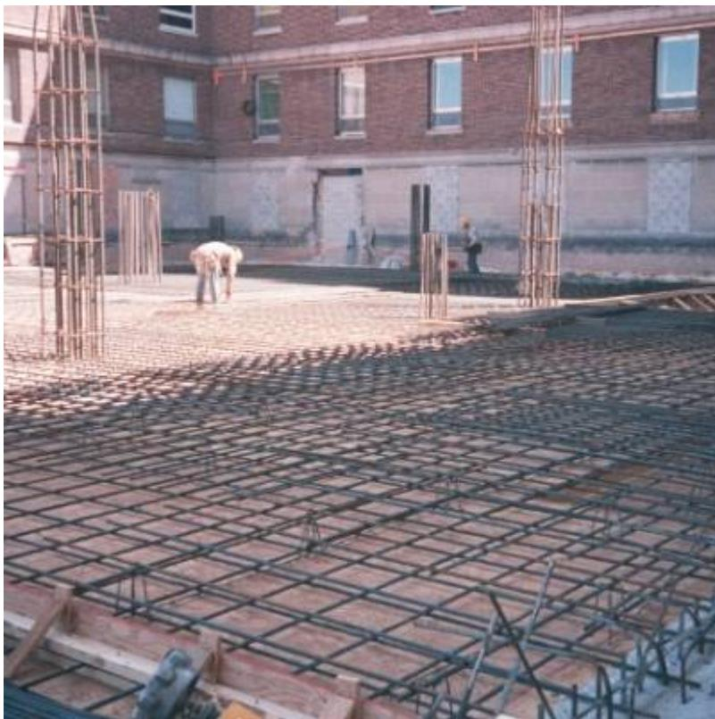
Fig. 22. Floor framing system - flat slab with drops.
