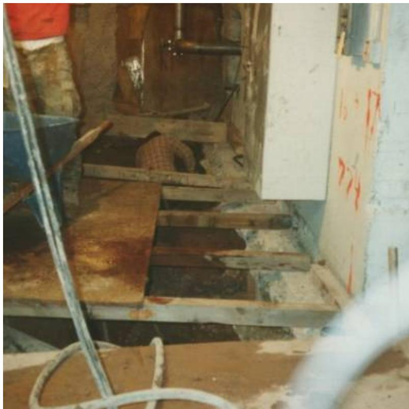
Fig. 8. Underpinning existing foundations.
