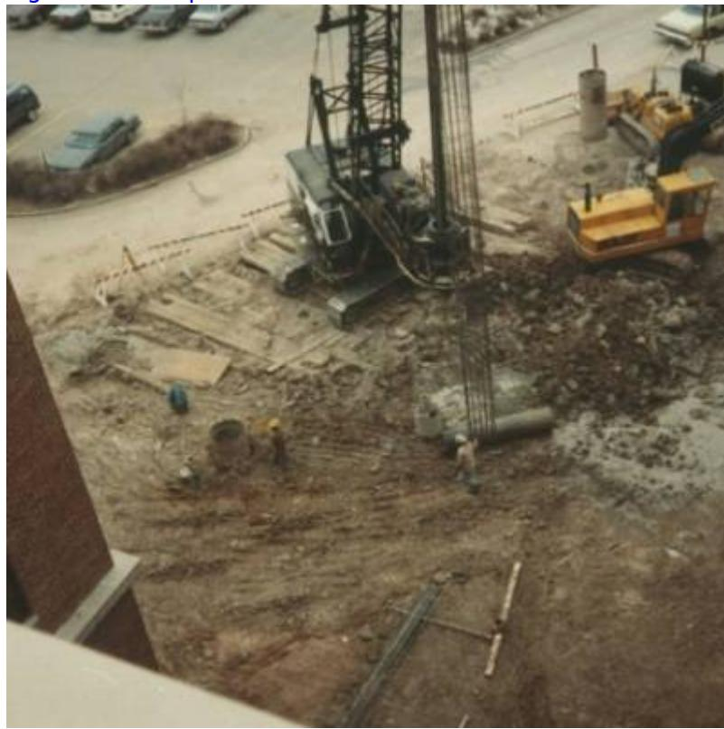
Fig. 13. Setting rebar cage in drilled pier.
