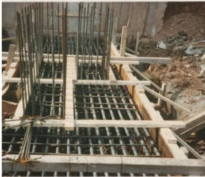
Fig. 19. Foundations - pier caps and grade beams.
