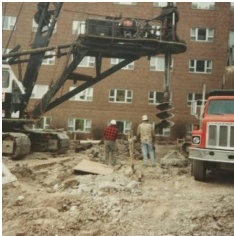
Fig. 12. Drilled pier installation.
