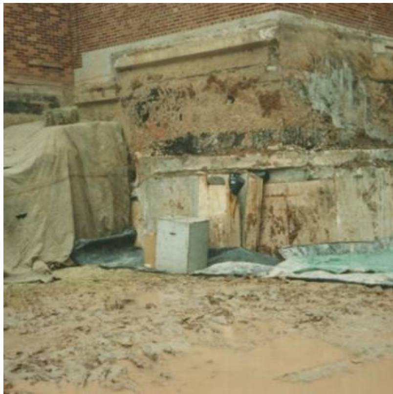
Fig. 9. Underpinning foundations for existing hospital pool.
