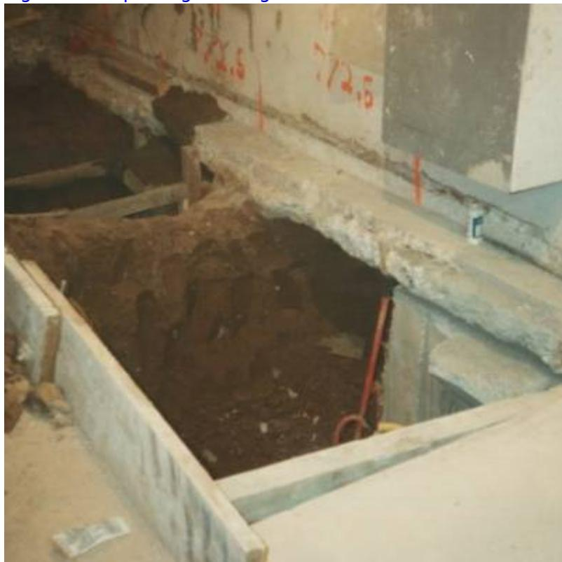
Fig. 8. Underpinning existing foundations.
