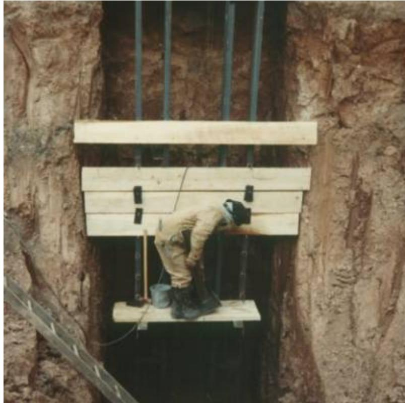
Fig. 7. Underpinning existing foundations.
