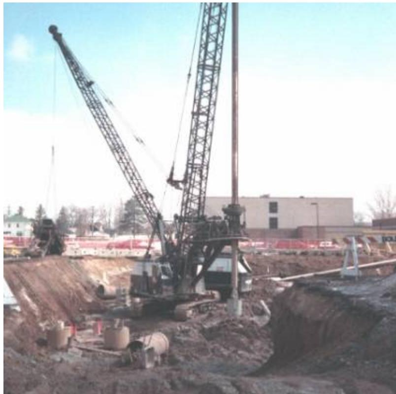
Fig. 11. Deep foundations utilized drilled piers.
