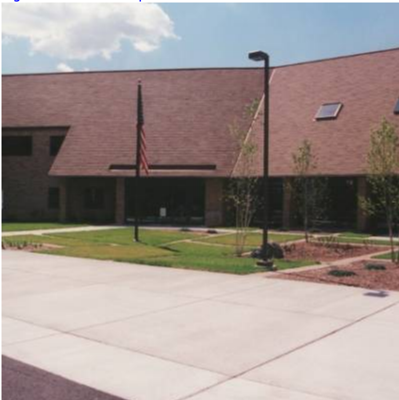
Fig. 3. St. Thomas Aquinas church and school addition.
