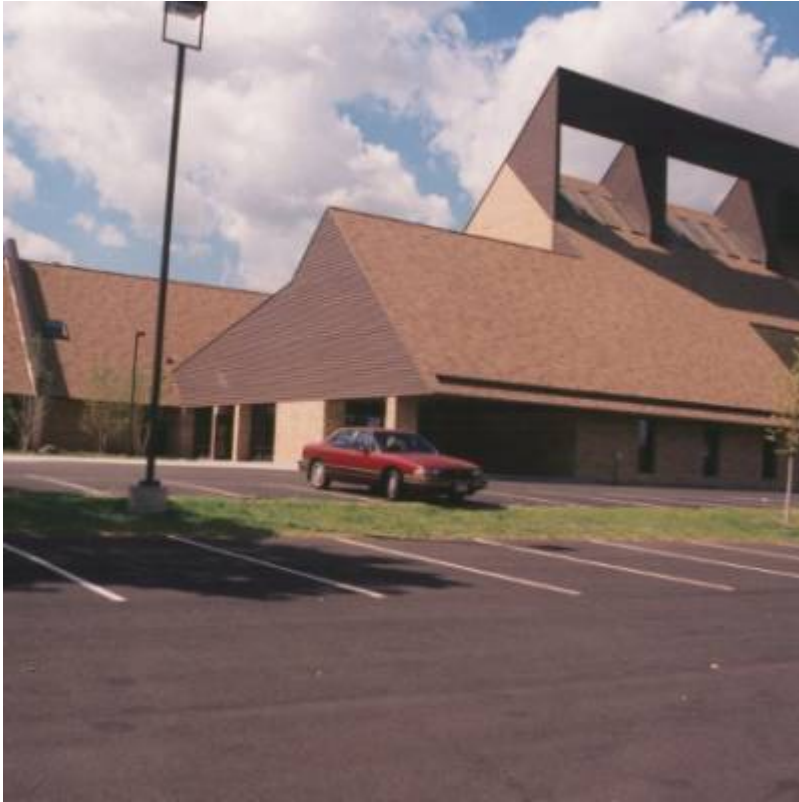
Fig. 4. St. Thomas Aquinas church and school addition.
