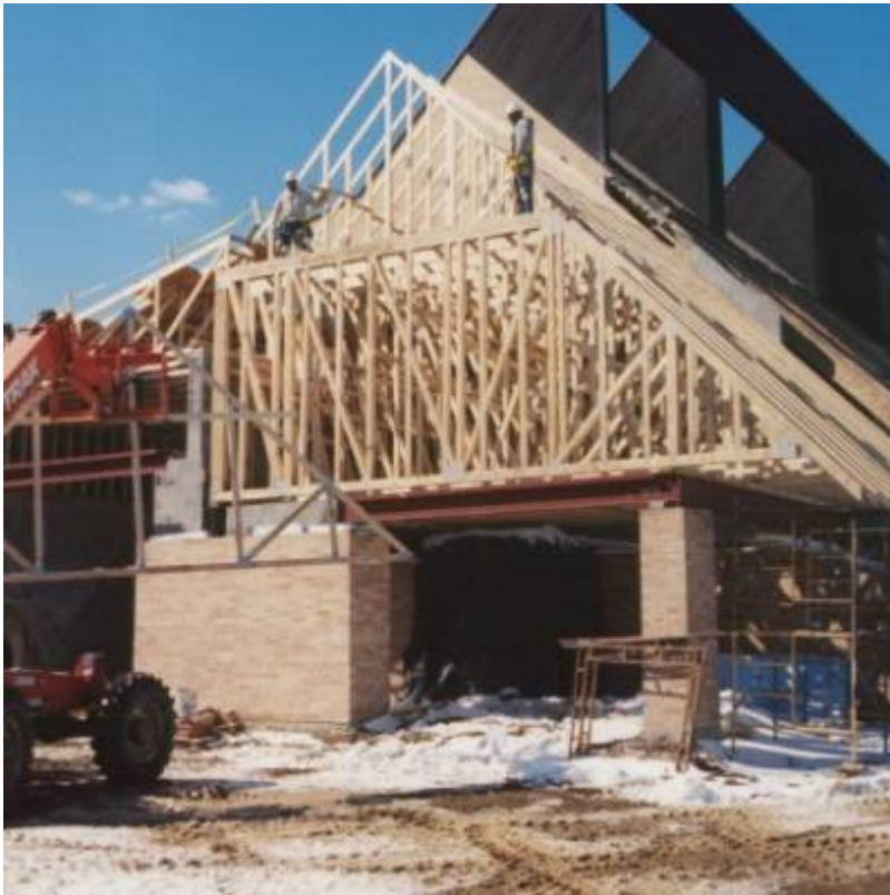
Fig. 2. St. Thomas Aquinas church and school addition.
