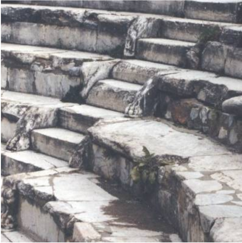
Fig. 5. The Odeion, noted detail at stairs.
