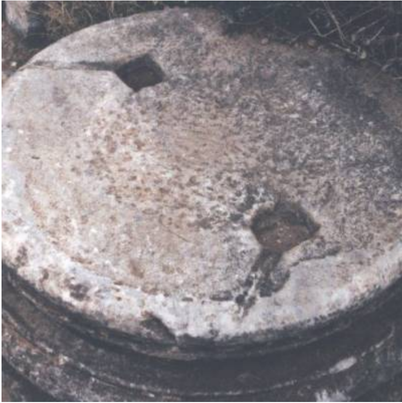
Fig. 9. Column base anchor detail.
