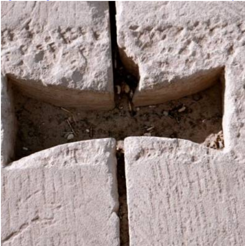
Fig. 11. Dovetail slot in wall of Kom-Ombo Temple.
