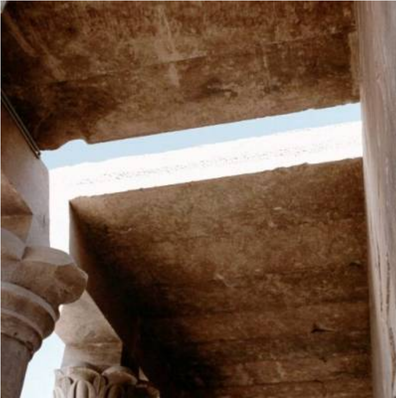
Fig. 5. Roof detail eastern colonnade.
