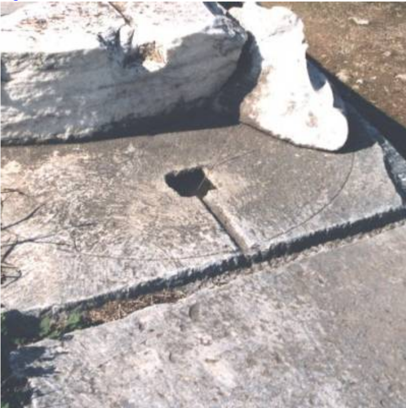
Fig. 6. Column base anchor detail.
