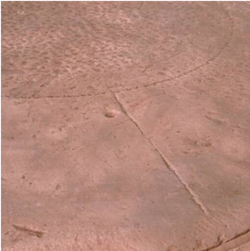
Fig. 2. Column base showing masons guide lines.
