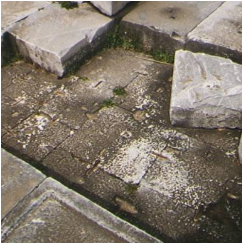
Fig. 8. Temple of Athena, paving anchor detail.
