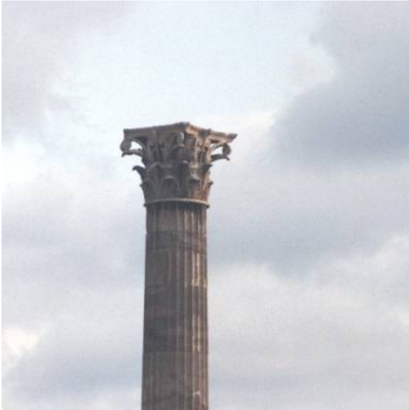
Fig. 3. Corinthian column detail.
