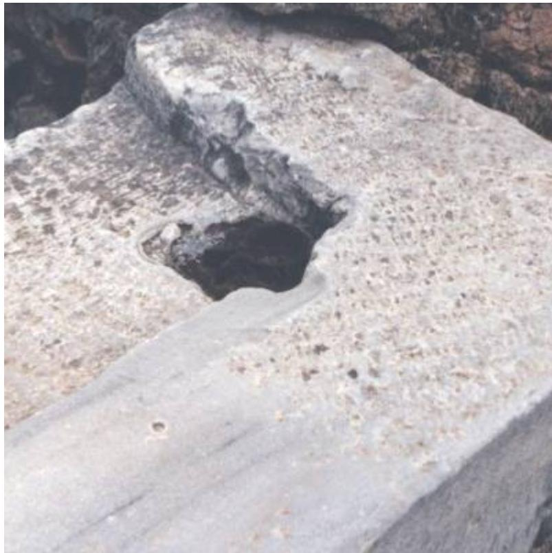
Fig. 7. Stone anchor detail.
