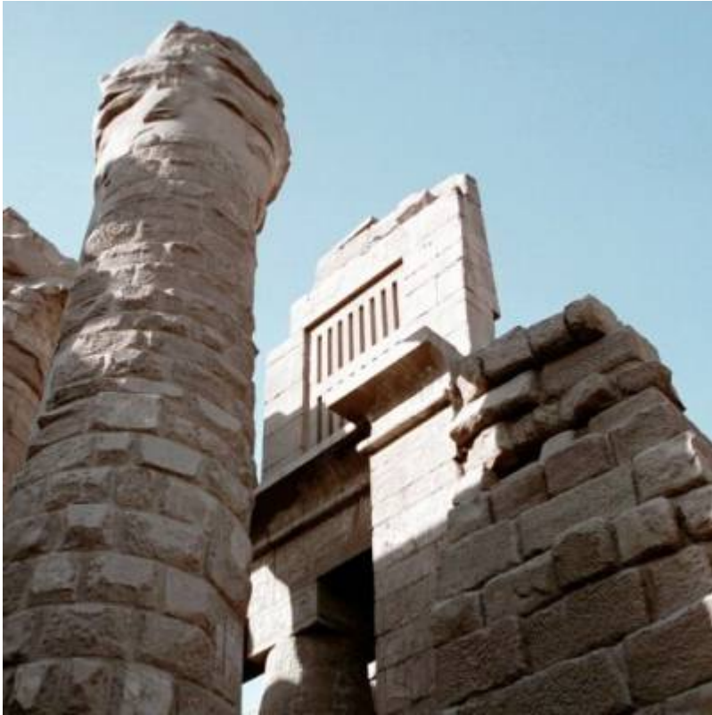
Fig. 11. Unfinished column and wall.
