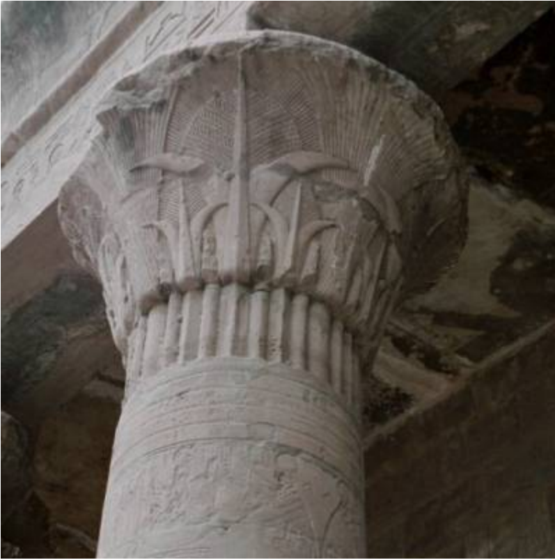
Fig. 6. Column capital detail from peristyle court.
