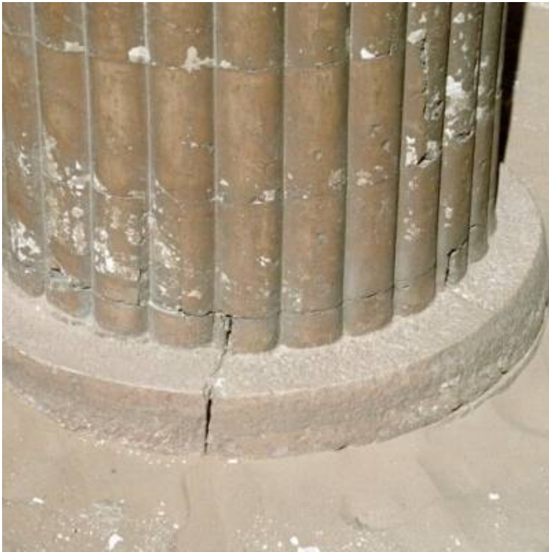
Fig. 5. Ribbed column-pilaster detail.
