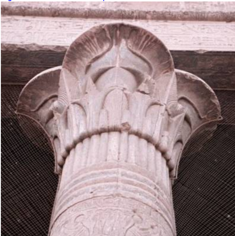
Fig. 4. Detail of column capital.
