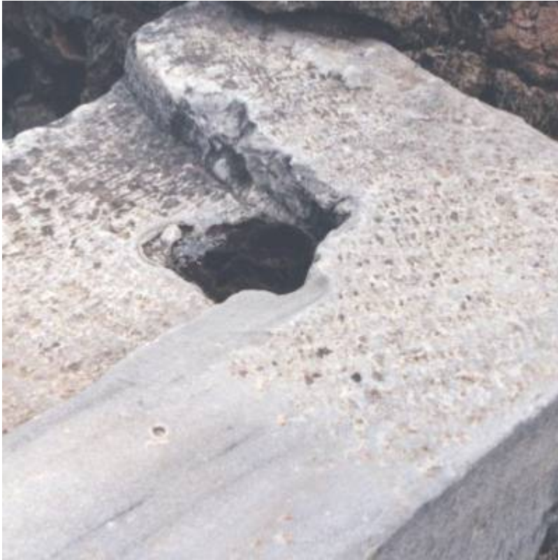
Fig. 7. Stone anchor detail.
