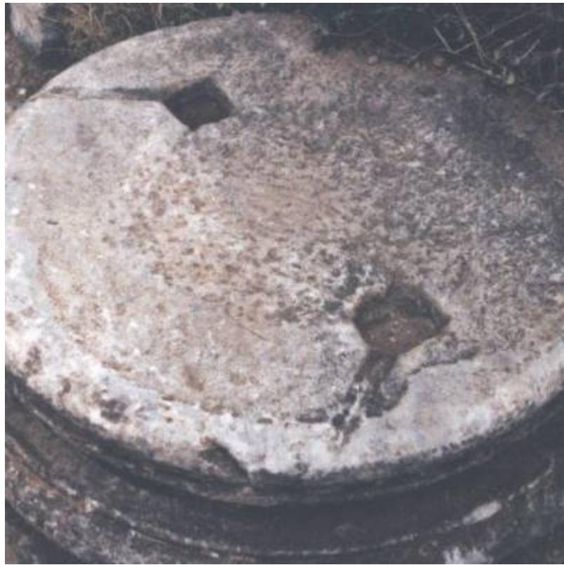
Fig. 9. Column base anchor detail.
