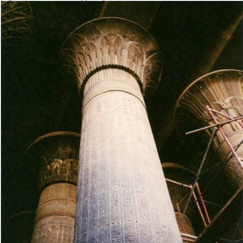
Fig. 6. Detail of column capital.
